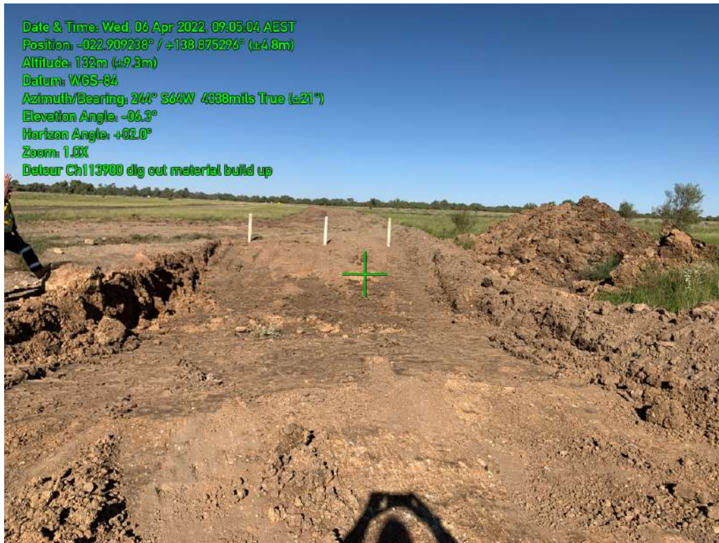
Figure 1 Donohue Hwy Detour Construction 2022 Works
