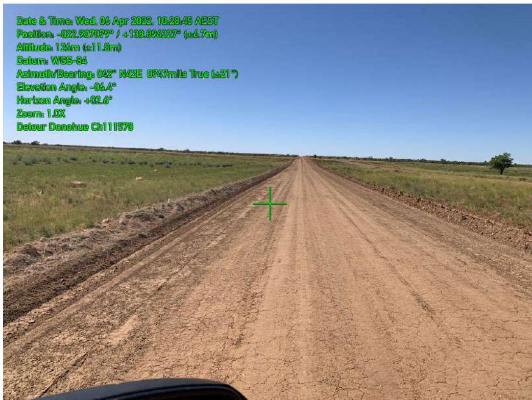
Figure 2 Donohue Hwy Detour Construction 2022 Works
