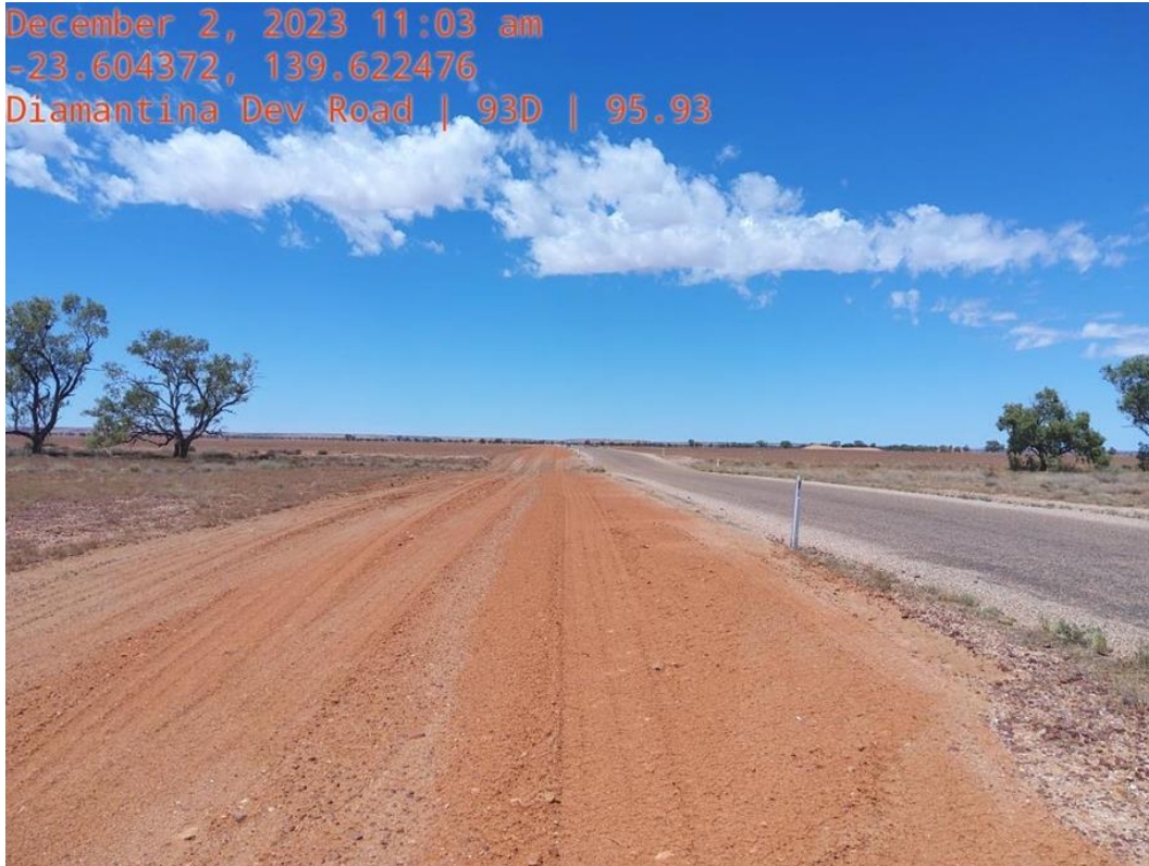
Bedourie Road - Bellview Flood Plain – Protection Works to existing Pavement - 93D
