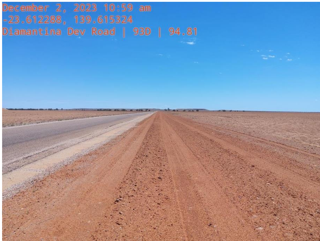
Bedourie Road – Protection Works to existing Pavement – 93D
