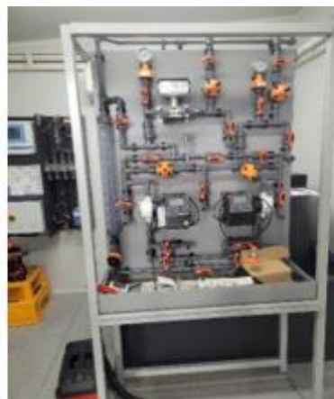
Existing Chlorination facility on skids to be removed from site. [Not refurbishing at this stage].
