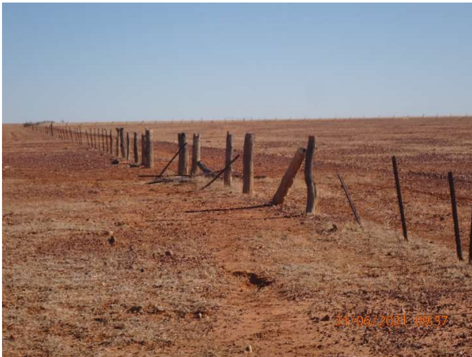
The Pony Club paddock/Kewpie boundary fence is in a sad state, it would be a fair to bad condition with broken/rotten off wood posts and broken wires.
