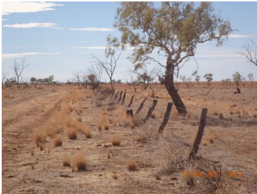
The Town Common fence on the Old Goodwood side of the Boulia/Winton Rd where the Town Common starts heading back to the Sandy Channels is fair to good with the odd broken wire and bent steel picket and broken wood except for the corner which needs some work/replacing.
