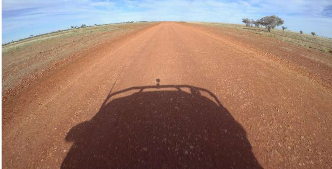
R2R South Urandangi Road Re-sheeting
