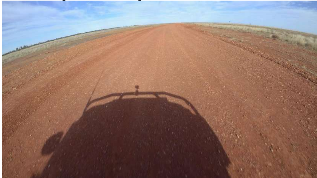
R2R South Urandangi Road Re-Sheeting
