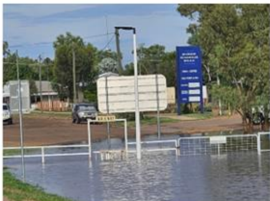
Boulia Road closed sign February 2024 River rising
