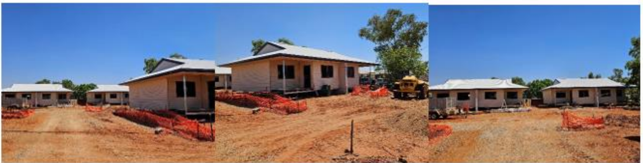
The building are near lockable stage.
